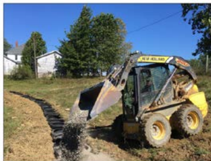
The tread cylinders are filled with rock.
