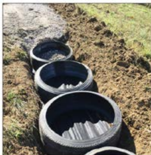
Nonwoven geotextile fabric and tread cylinders are placed in a trench and backfilled with dense-grade aggregate (DGA).
